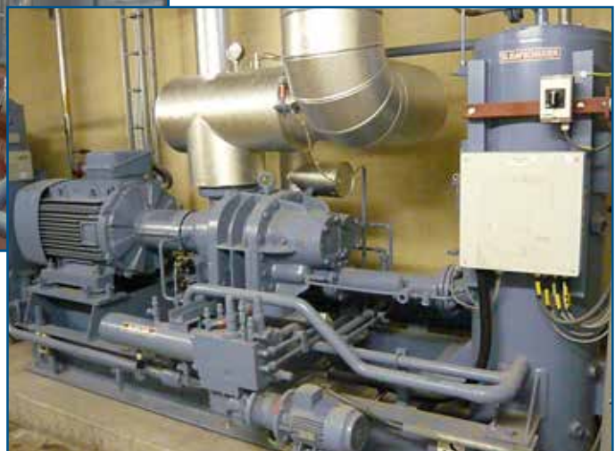
Screw compressor for refrigeration
