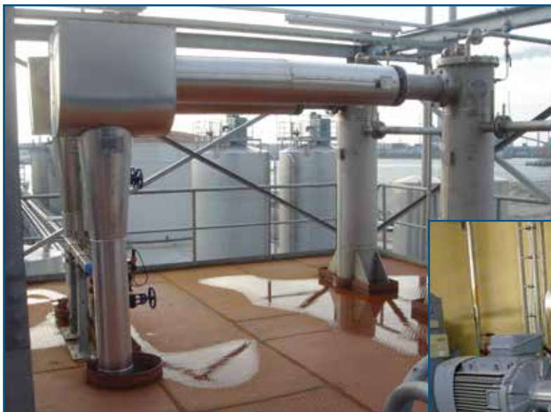
2-stage steam jet vacuum ejectors with shell and tube condenser
