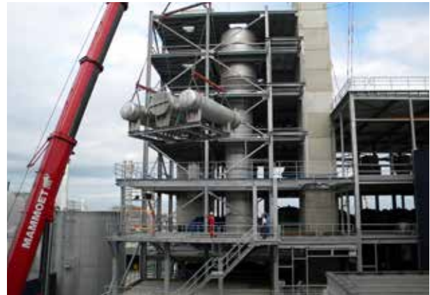
Assembly of an ice condensation block at site
