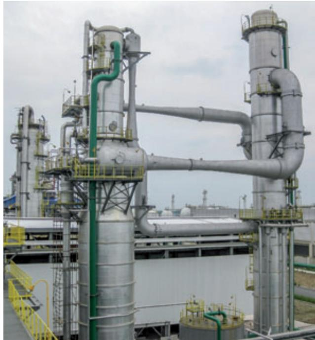
Free-standing construction: without secondary steel construction.
